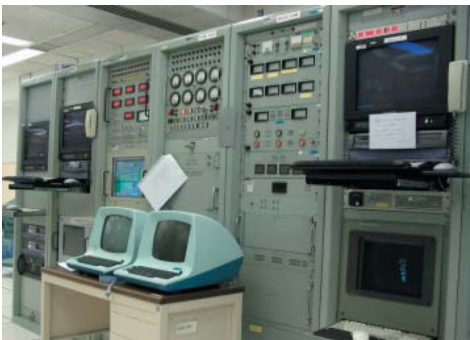
Receiver racks for the 70 m antenna (DSS-63) in the Signal Processing Center from where all raw data is sent to the Jet Propulsion Laboratory for interpretation. P. Corneille
